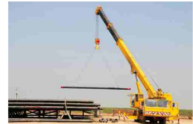
Lifting and Heavy Equipment
